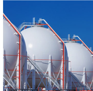
Major Hazards Page 20
